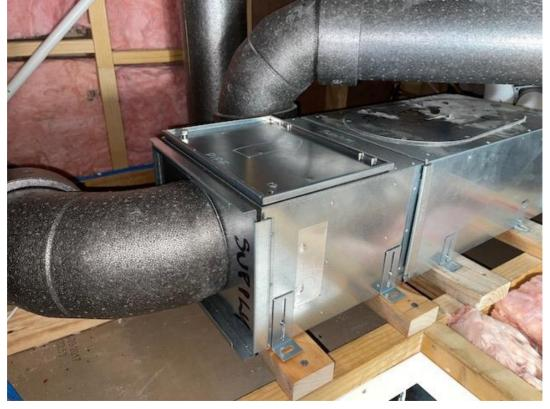
I chose to install the housing just next to the manhole and directly to the attenuator. The screws (by hand) can be undone to flip the hinged 'lid' exposing the filter to install or remove.
